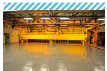
High-level vitrified waste storage hall – La Hague facility
