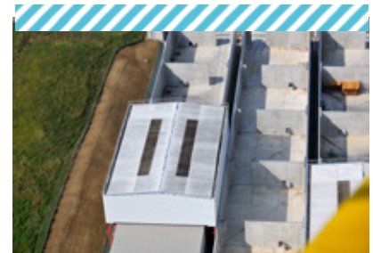
Aube disposal facility – vaults being filled
